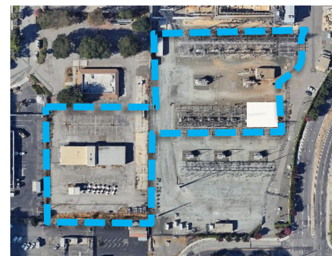
Kifer Receiving Station
