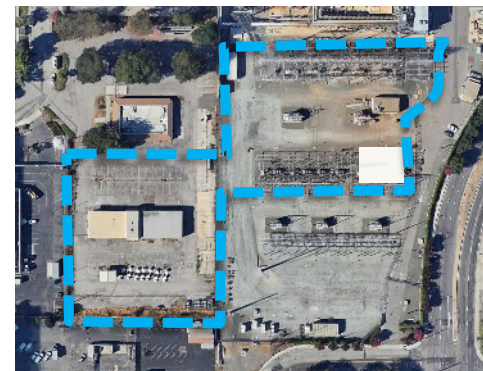
Kifer Receiving Station
