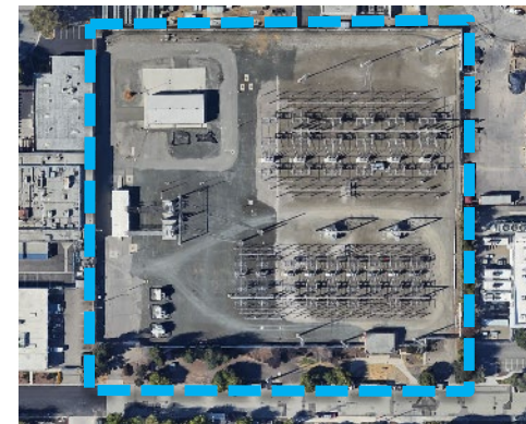
Scott Receiving Station
