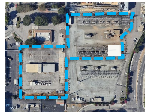
Kifer Receiving Station
