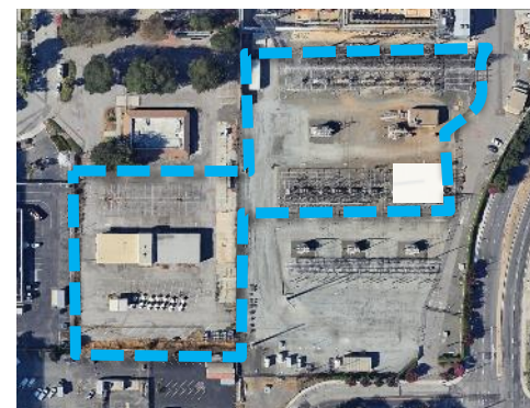
Kifer Receiving Station
