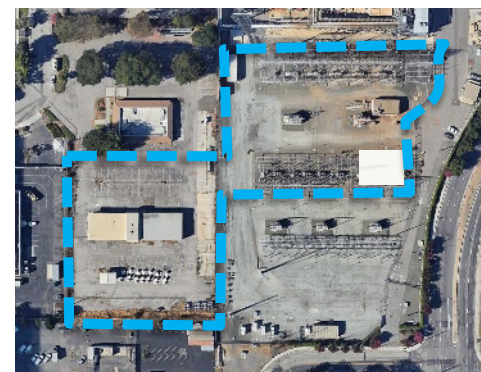
Kifer Receiving Station
