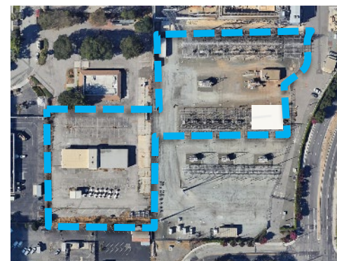
Kifer Receiving Station
