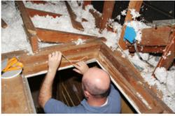
**Attic access hatches are rarely weather stripped, leading to significant air leakage around the edges of the access hatch.**
