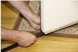
**Once you have a new door shoe (or have confirmed that the existing one is in good condition), slide it into the threshold bracket.**
