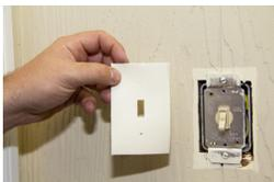
**Light switches and outlets on exterior walls are a common location of air leakage.**
