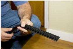
**One of the best solutions for stopping air leaks at the bottom of a door is a door shoe.**
